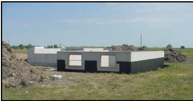
The foundation has been poured in Emery.
