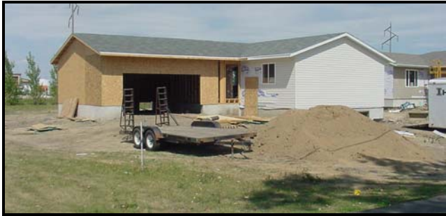
The house in Alexandria (windows will be added soon).
