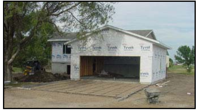
Preparing for siding on the Plankinton Vine Street site.
